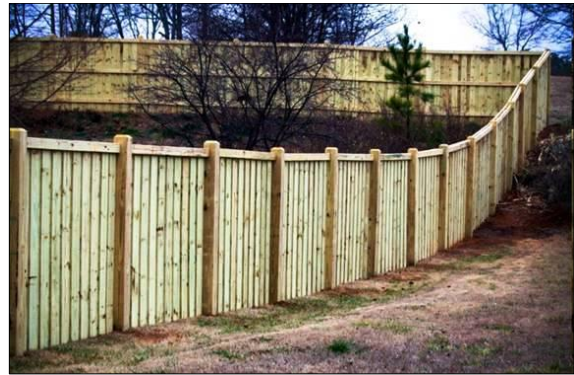
Figure II-14: Fence Finished Side Example
